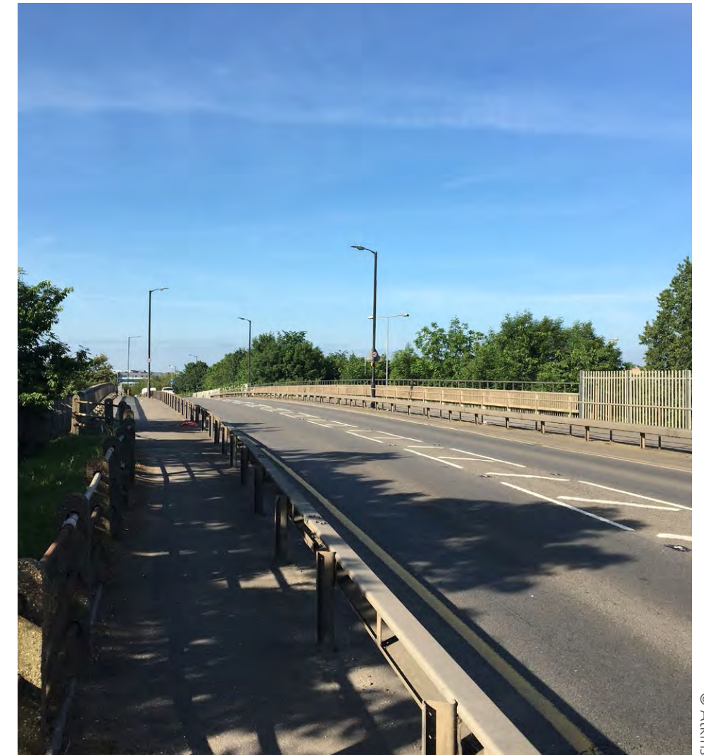
Existing bridge over M4
