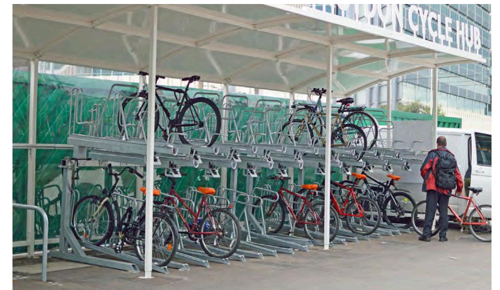
Cycle hub at stations
