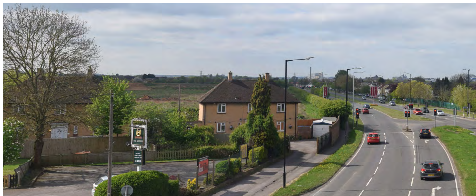
View looking south towards former nursery which is in the process of being excavated for gravels
