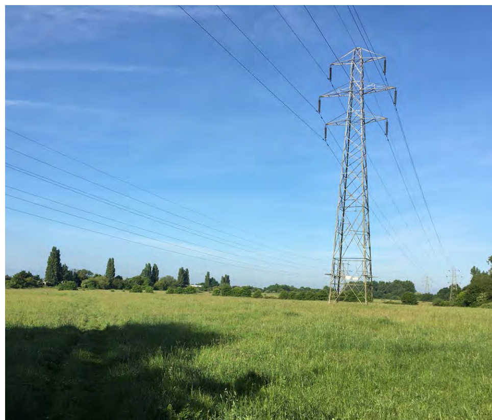
Overhead powerline running to the south of Orchard Park
