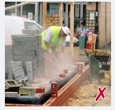
▲ No measures are being taken to control the dust generated by the use of this disc cutter. Workmen and others will be inhaling the damaging dusts.
