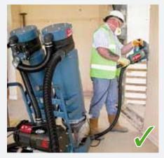
▲ Dust extraction equipment fitted to the tools can be used to control silica dust where the use of water is not practicable.
