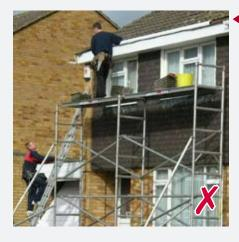
Tower scaffolds and ladder platforms should not be used without guard rails when replacing gutters etc. Assembly instructions provided with towers should be followed.
