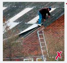
This workman is at risk of falling through the roof, through a roof light or from the roof edge. The ladder access is unsecured and too short. Walking along the line of the purlins (roof supports) is not acceptable.
