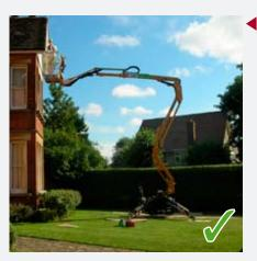
Work from ladders can be undertaken more safely from a tower scaffold or a mobile access platform.Towers and mobile access platforms should be erected and used by competent people.
