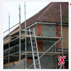
Guard rails are missing from this scaffold. Scaffolding must be erected by competent people, to a recognised standard, properly maintained and inspected regularly.
