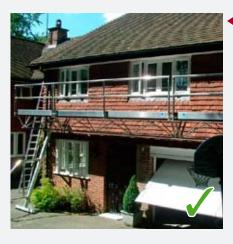
This photograph shows a properly erected proprietary working platform. Such system scaffolds should be erected in accordance with the suppliers instructions.
