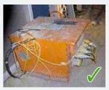
Photograph shows a 110v (centre tapped to earth) electrical supply from a transformer commonly used on construction sites to reduce the risk of electrocution.
