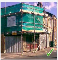
A well-constructed scaffold is based on solid foundations and fitted with guardrails, toe boards and bracing. It must be tied to the building unless designed to be free standing. This also shows use of netting to prevent falls of material.
