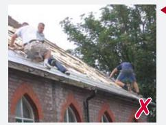
These men are re-roofing a sloping roof without edge protection to prevent falls. This is highly dangerous.
