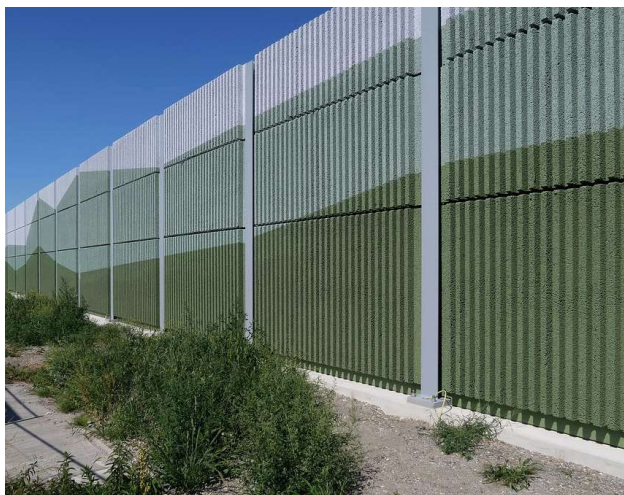
Figure C6.4.1: Examples of roadside acoustic fencing
