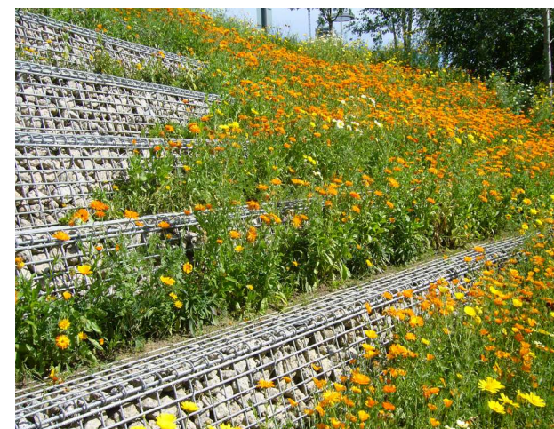
Figure C5.1.4: Retaining structures - gabion baskets
