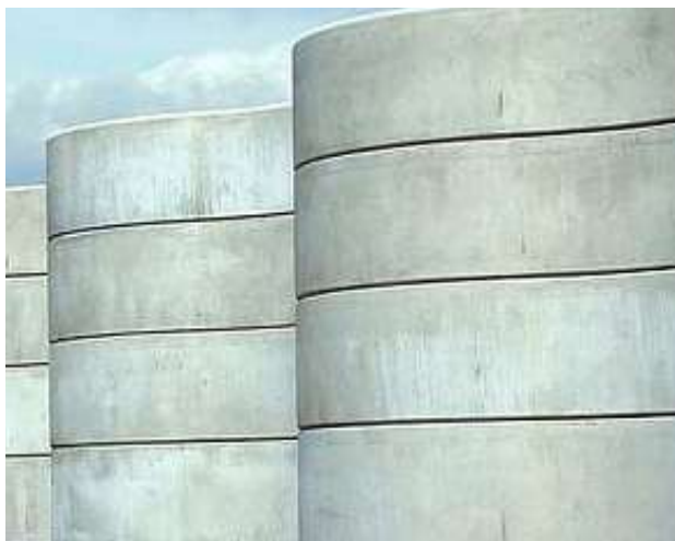
Figure C6.3.3: 5m high freestanding blast walls at T5
