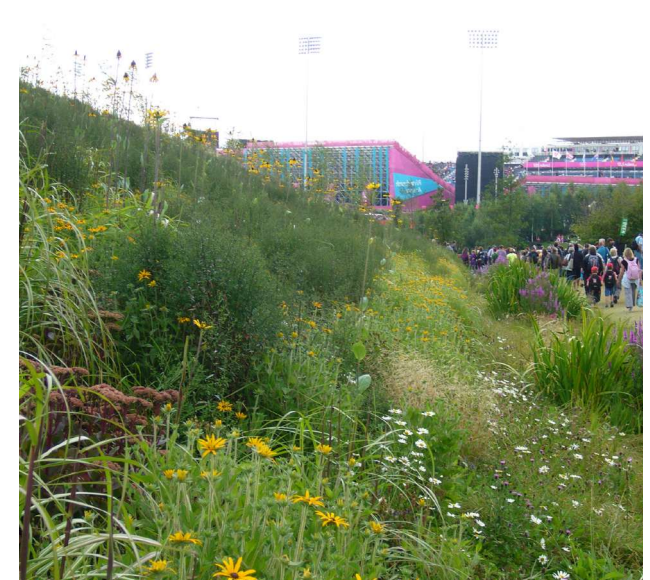
Figure C5.2.4: Temporary bunds for visual mitigation
