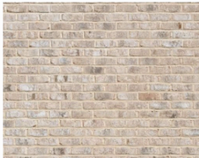
Recycled brick on the office facade
