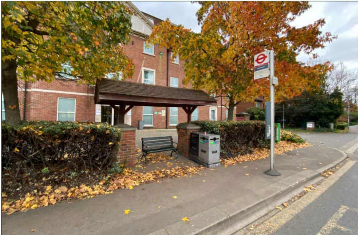
Photo 2-4: Poyle Road Junction Eastbound Bus Stop
