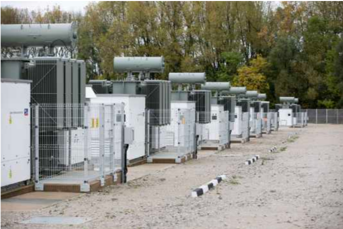
Indicative image of a typical BESS
