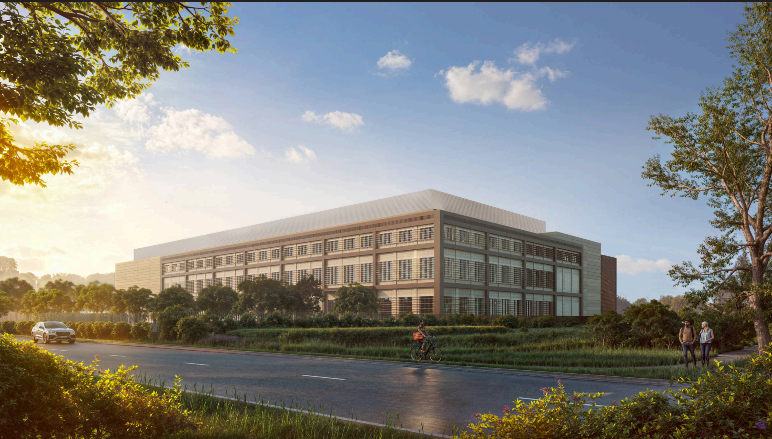
View to the Data Centre building, looking north-west from the main access.
