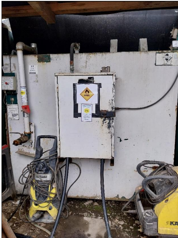
Photo 15: An externally located 8,500 L diesel tank in A S Transport with staining observed beneath.
