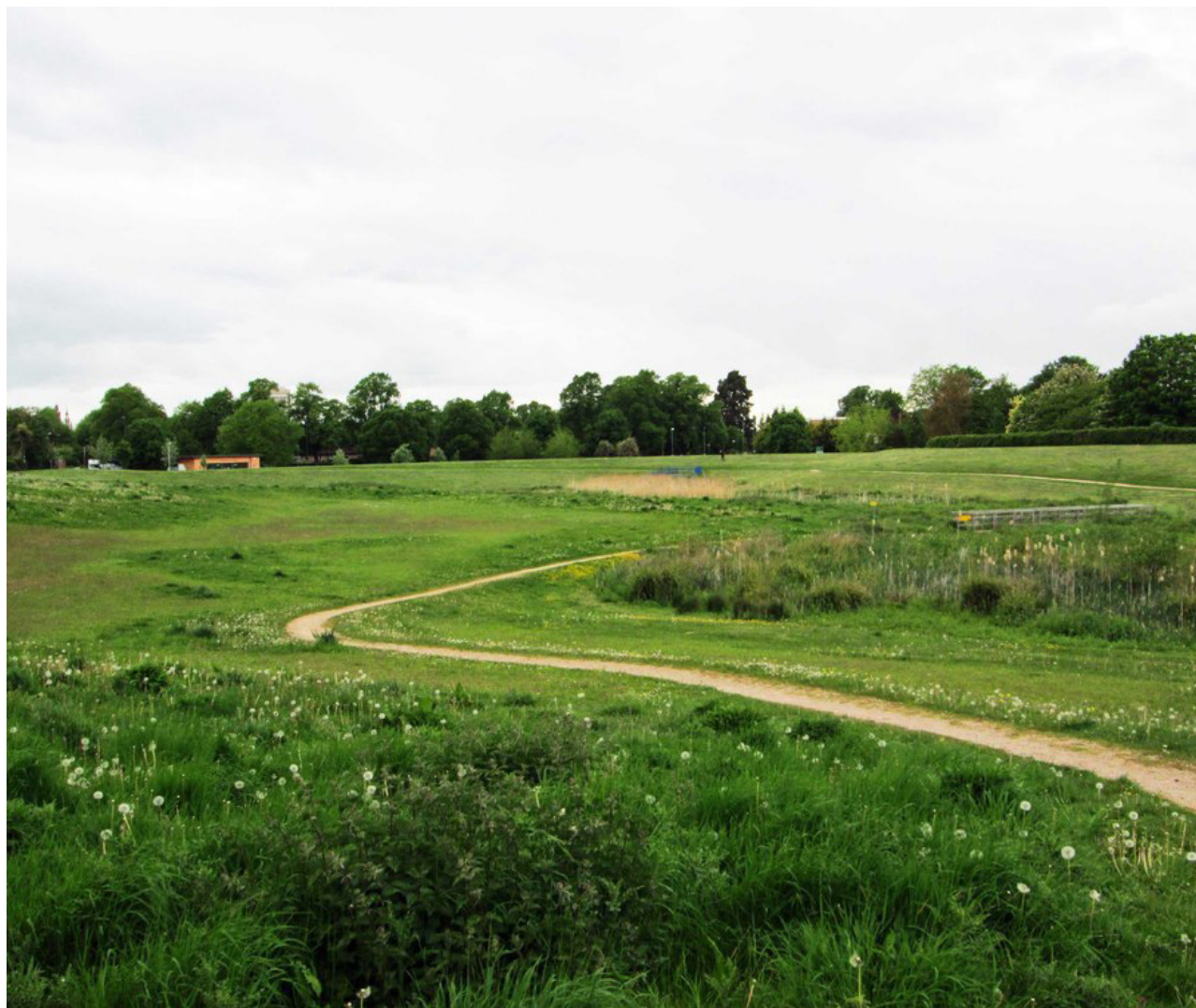
Figure C2.2.2: Example of dry storage basin
