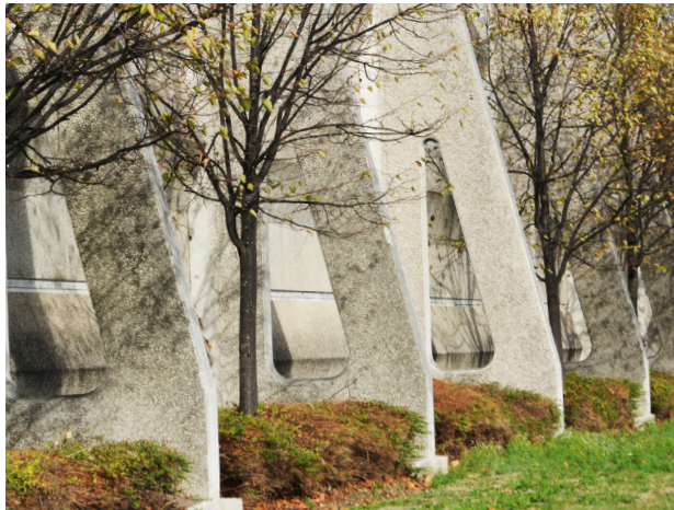
Figure C6.3.1: Planted blast walls along the Southern Perimeter Road
